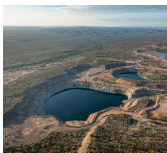
Figure 12: Kidston pumped hydro reservoirs
