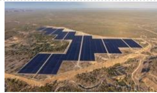
Jemalong Solar Project 50MW Solar Project
