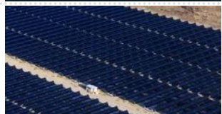
K2-Solar Up to 270MW Solar Project
