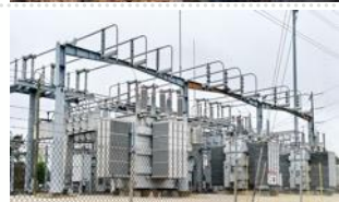
Bouldercombe Battery Project 50MW Large Scale Battery Energy Storage System
